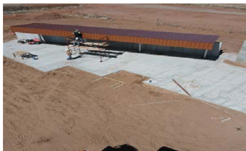
Installation of the shade canopy
