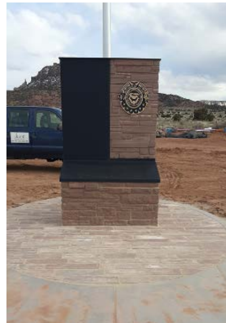
Right: Installation of flagstone at Zuni Monument using flagstone salvaged from the demolition of the old Senior Center
