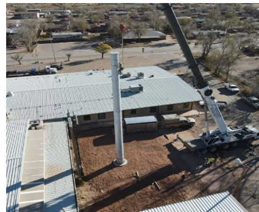
Installation of the 60-foot cell tower at the Tribal Administration building
