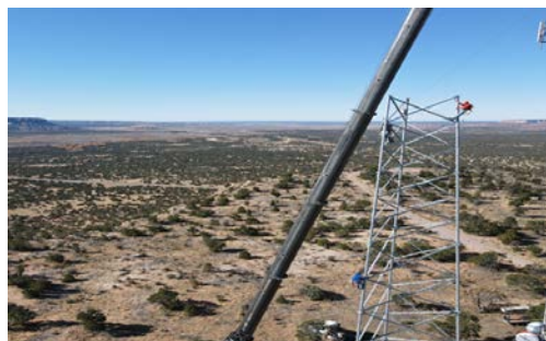
Installation of the 198-foot tower at the ridge site
