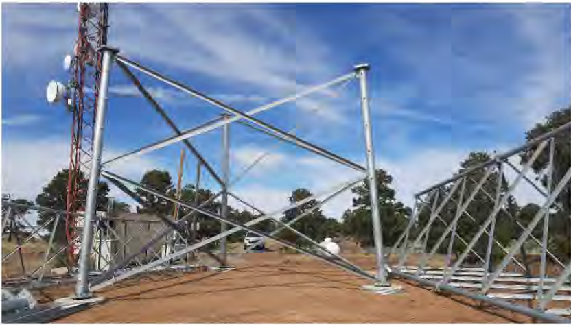
New, 198-foot cell tower under construction above Route 4
